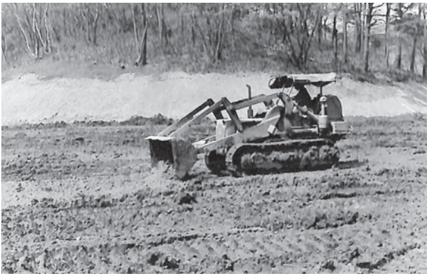
fig.10 「児童遊園盛土作業中及び地均し」1966年、「児童館児童遊園工事写真」スクラップブック、文化庁国立近現代建築資料館 17-3-1-17 〈Banking and Leveling in the north-west part of the Kodomo No Kuni Playground〉 1966, From the album of document photos of construction of the Kodomo No Kuni playground. National Archives of Modern Architecture, Agency for Cultural Affairs, inv. 17-3-1-17
